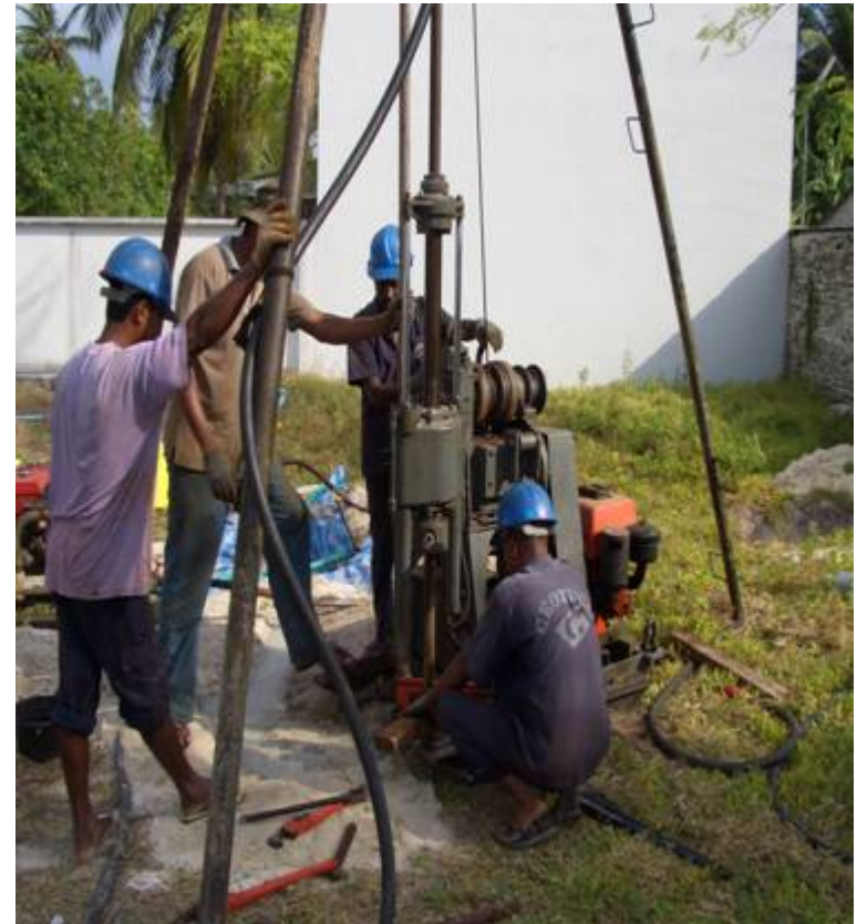
Drilling the 2 x 10m bore holes
