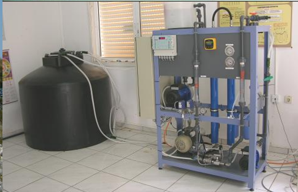
PV-Wind RO unit installed by CRES in Greece
