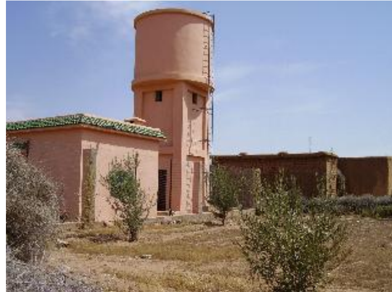
View of the water point
