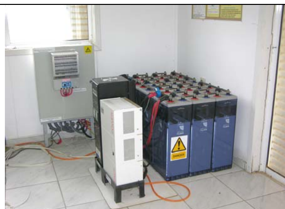
Pic. 30 The battery bank, the inverters and the chargers of the autonomous system
