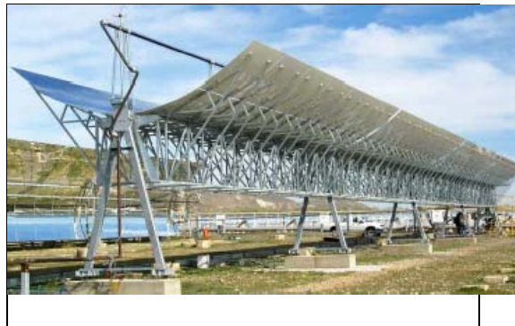
Pic 39 The EuroTrough collector prototype tested at PSA has currently four, later six - collector elements to one side of the hydraulic drive
